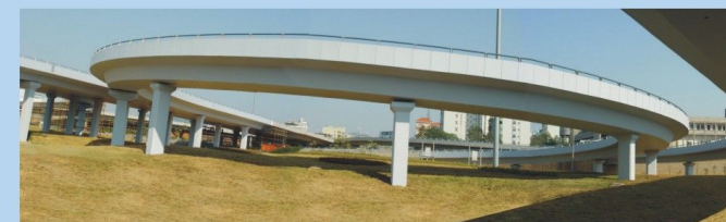
Liuzhou Shengli Viaduct, China
