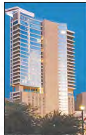
Completed structure with monostrand and bonded multistrand systems.
