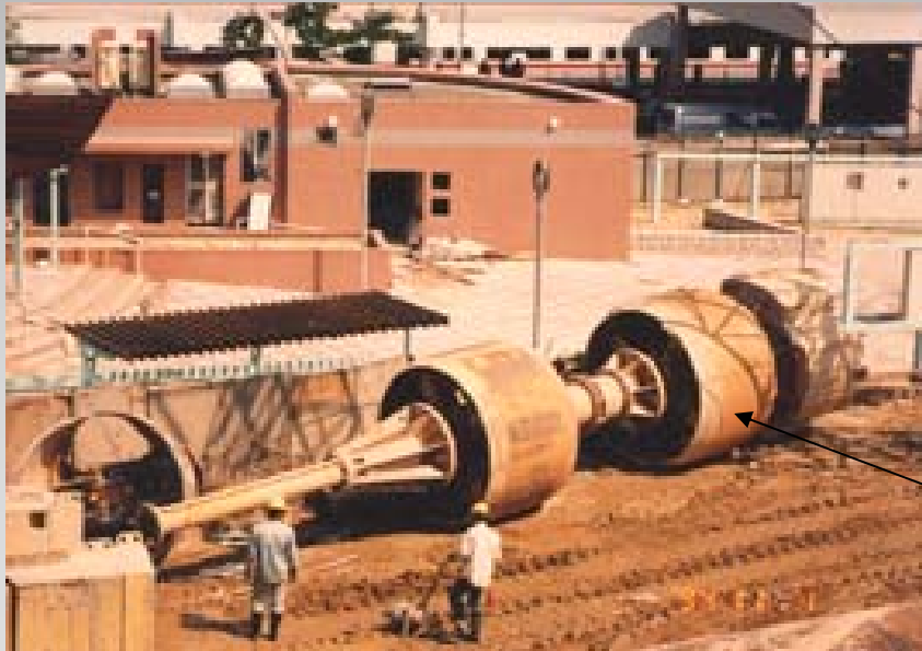
The set-up – RCD rig, serving crane and spoil separating tank
