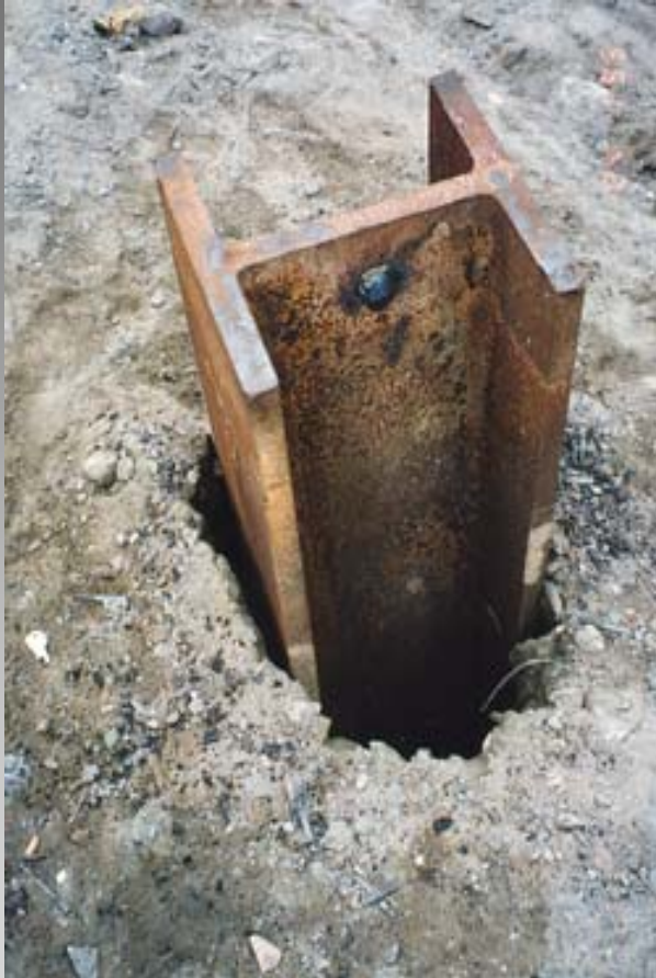
Inserting H-pile after pre-boring
