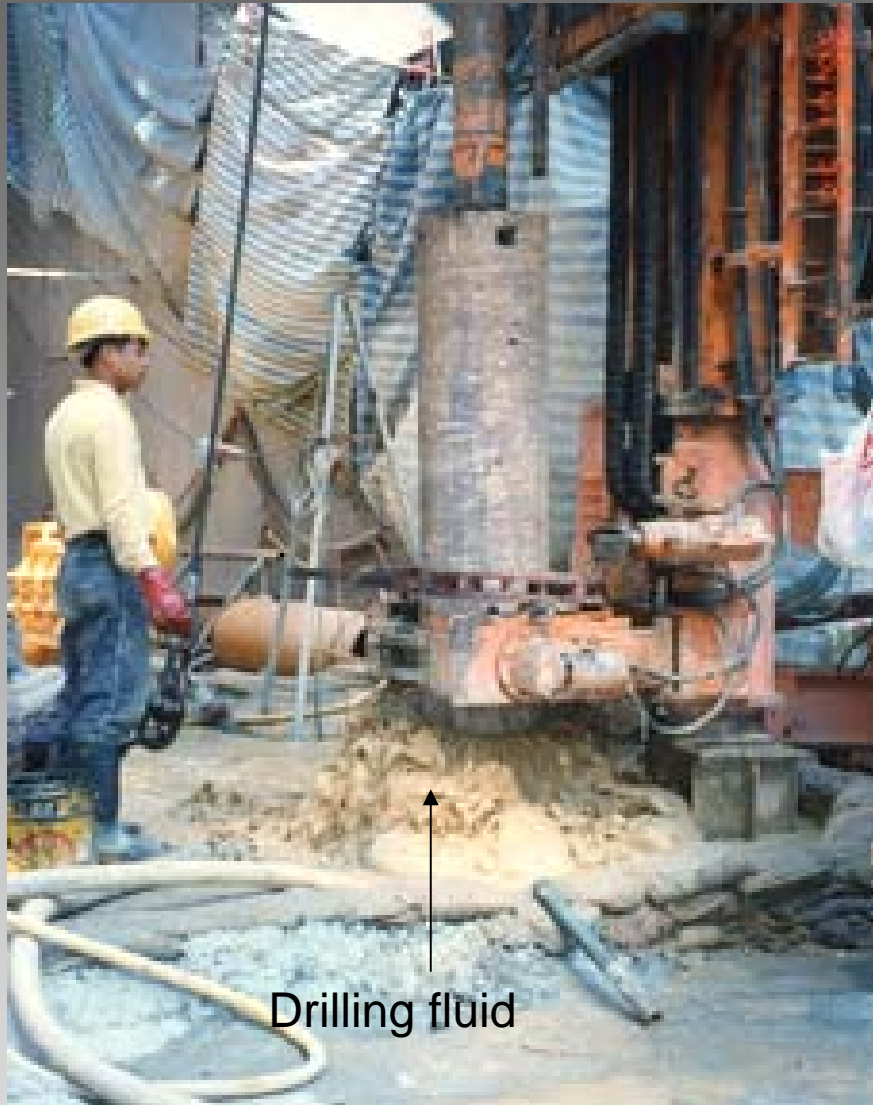
Using of drilling fluid to remove mud from bore hole
