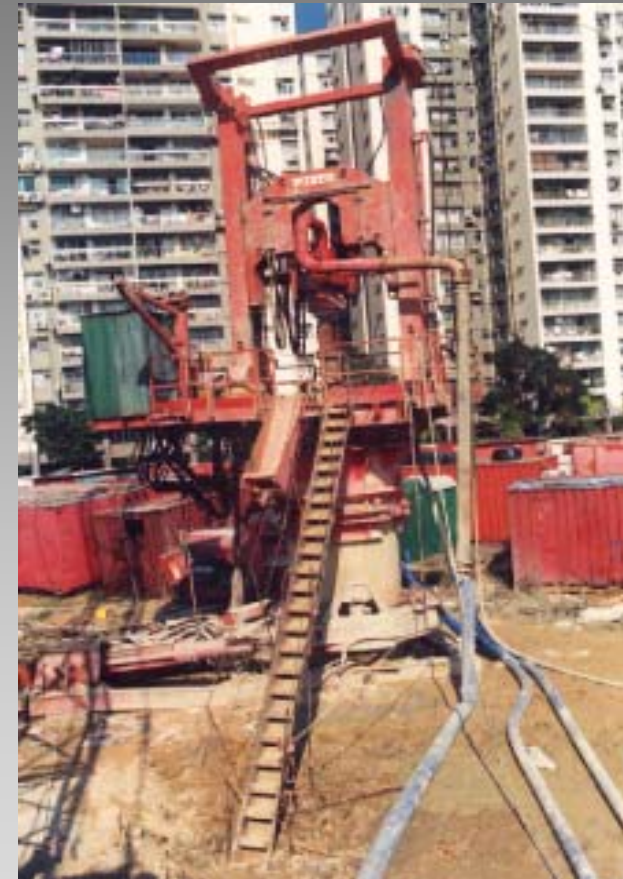
Large dia. Pile formed by reverse circulation drill
