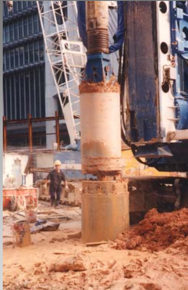
Bucket barrel taking soil from the borehole
