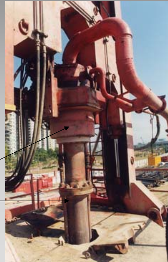
The rotating shell for driving the drilling rod
