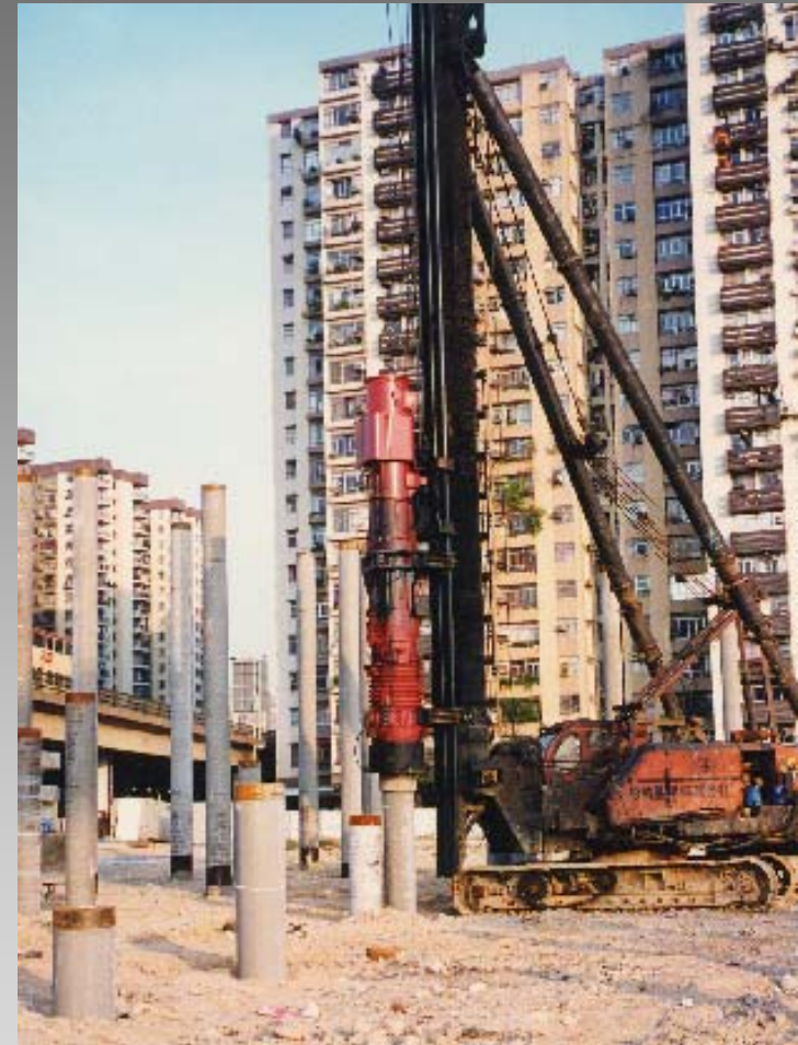
Precast circular-section pile driven by diesel hammer
