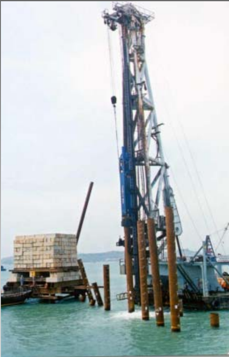
Piles for marine facilities
