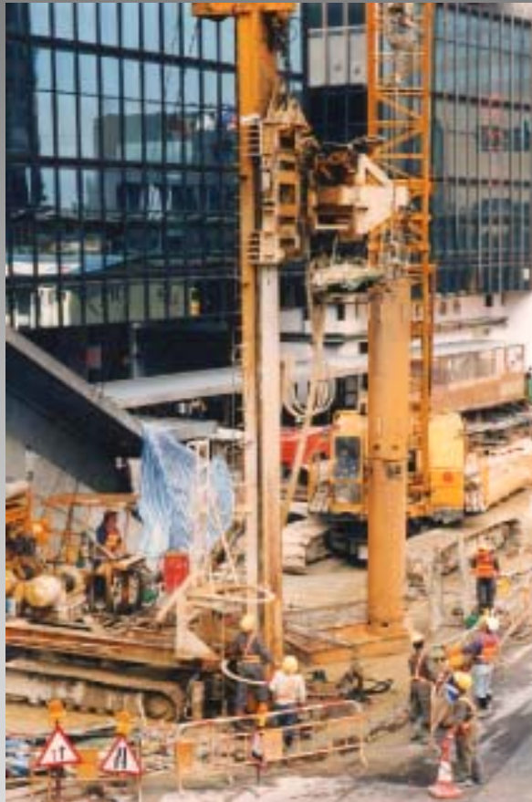
Small dia. pile formed using boring rig and drill
