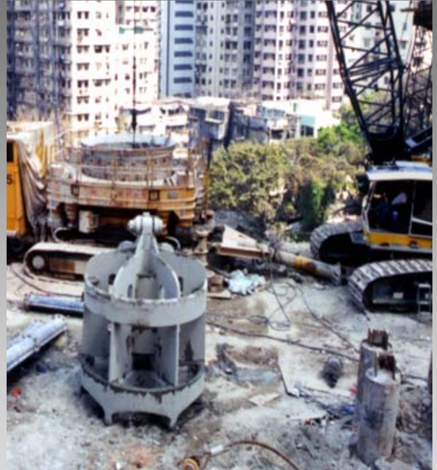
Various forms of chisel (for rock breaking)
