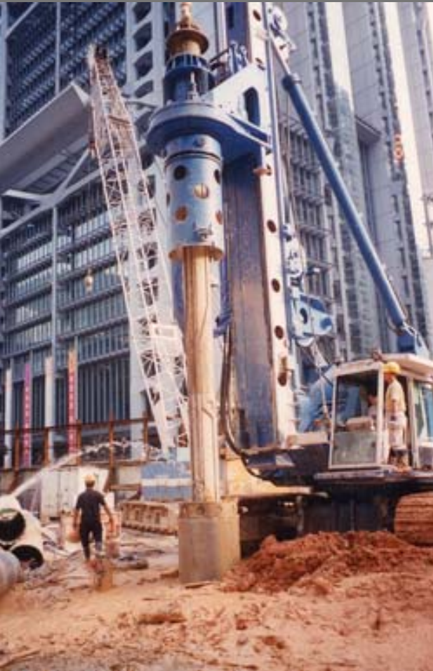
Bucket barrel taking soil from the borehole
