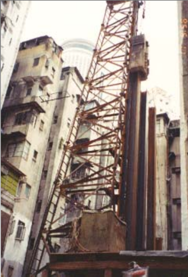
H-pile driven using gravity drop hammer
