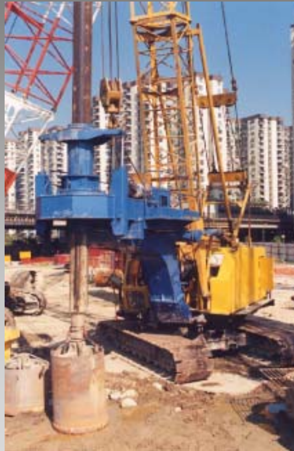
Medium dia. pile formed using bucket barrel
