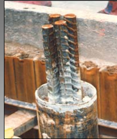
Detail of the inserting bars and the grouted pile
