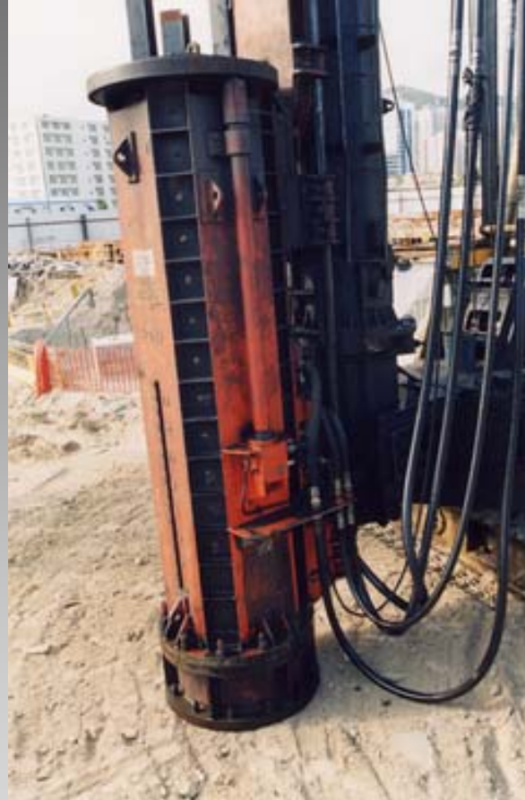
Hydraulic hammer for driving pile
