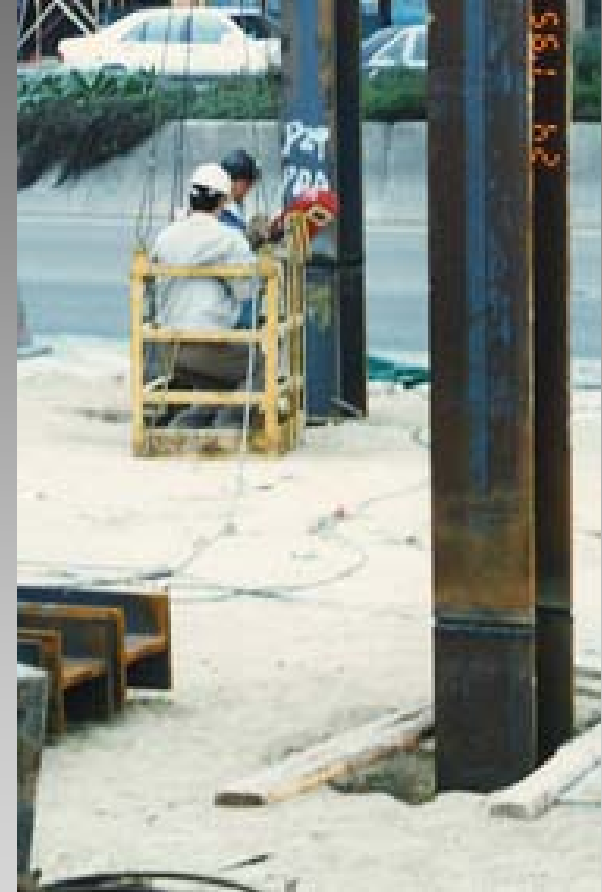
Site welding to connect H-piles (12m per pile)
