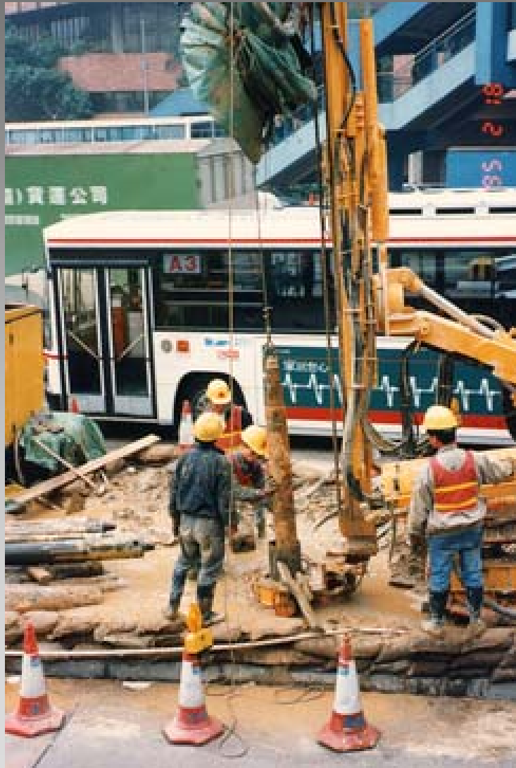
Driving mini-pile using compact-size drilling rig in congested environment
