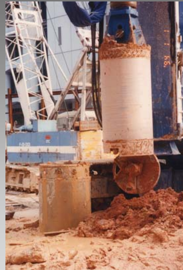
Bucket barrel taking soil from the borehole
