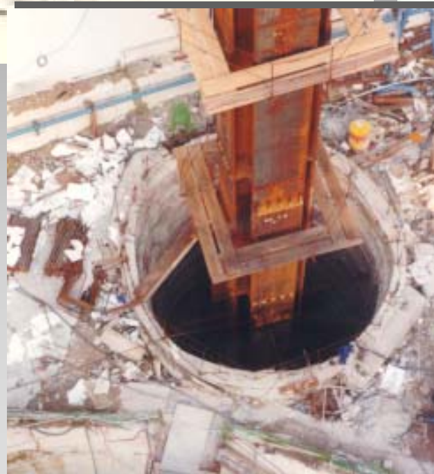
A 6.5m dia. caisson/ cofferdam for the insertion of a super- column (Cheung Kong Center)
