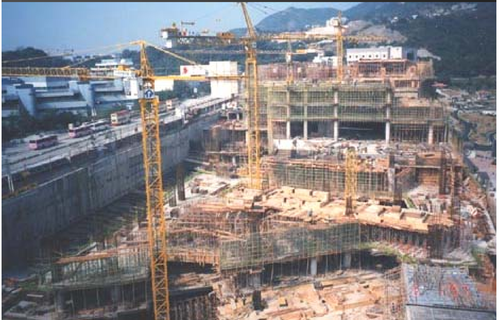
Construction of the superstructure and the top-down basement at its peak
