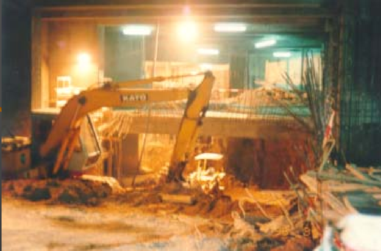
Excavation inside the top-down basement
