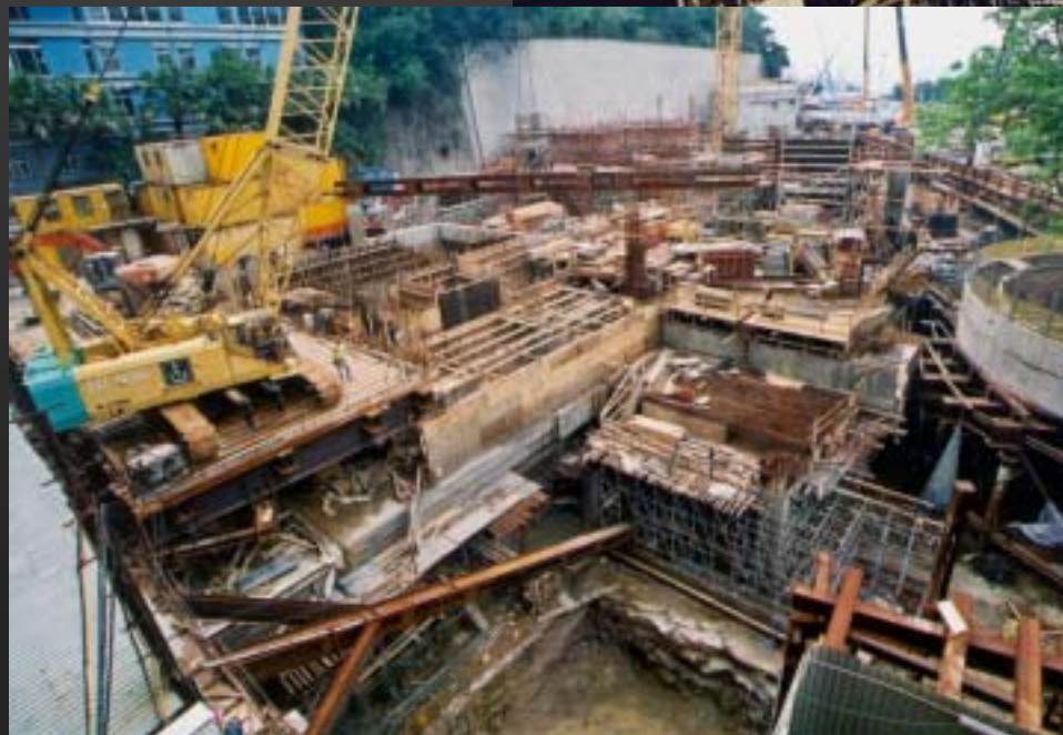
Construction of the TST East Station, KCR East Rail TST Extension
