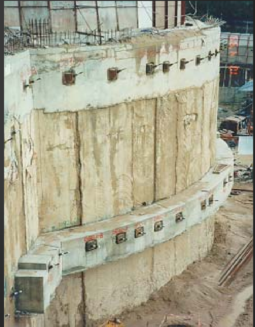
Using ground anchor
