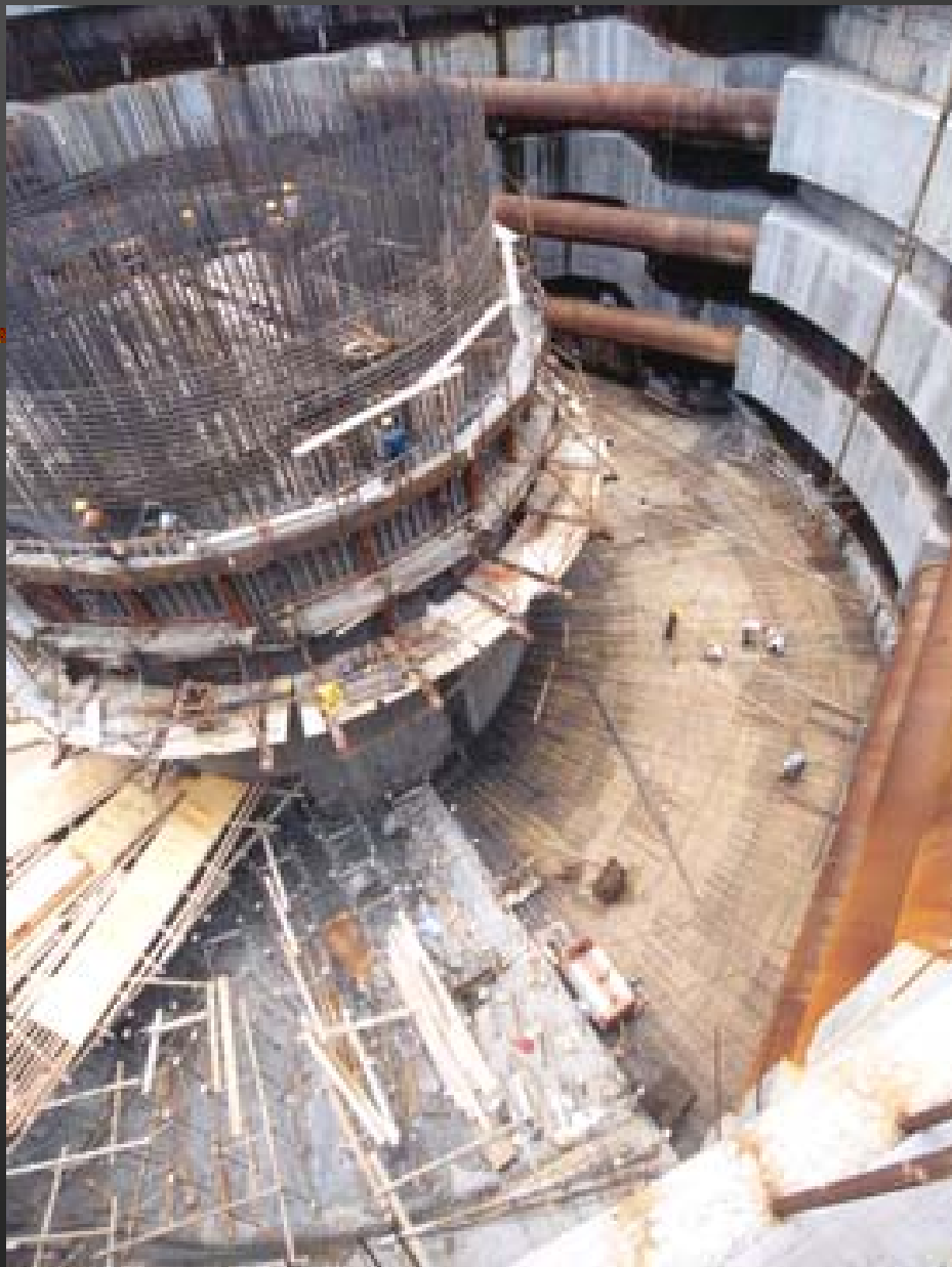
Forming the circular ramp
