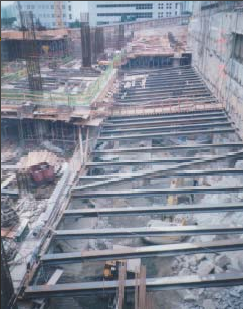
Using steel strut
