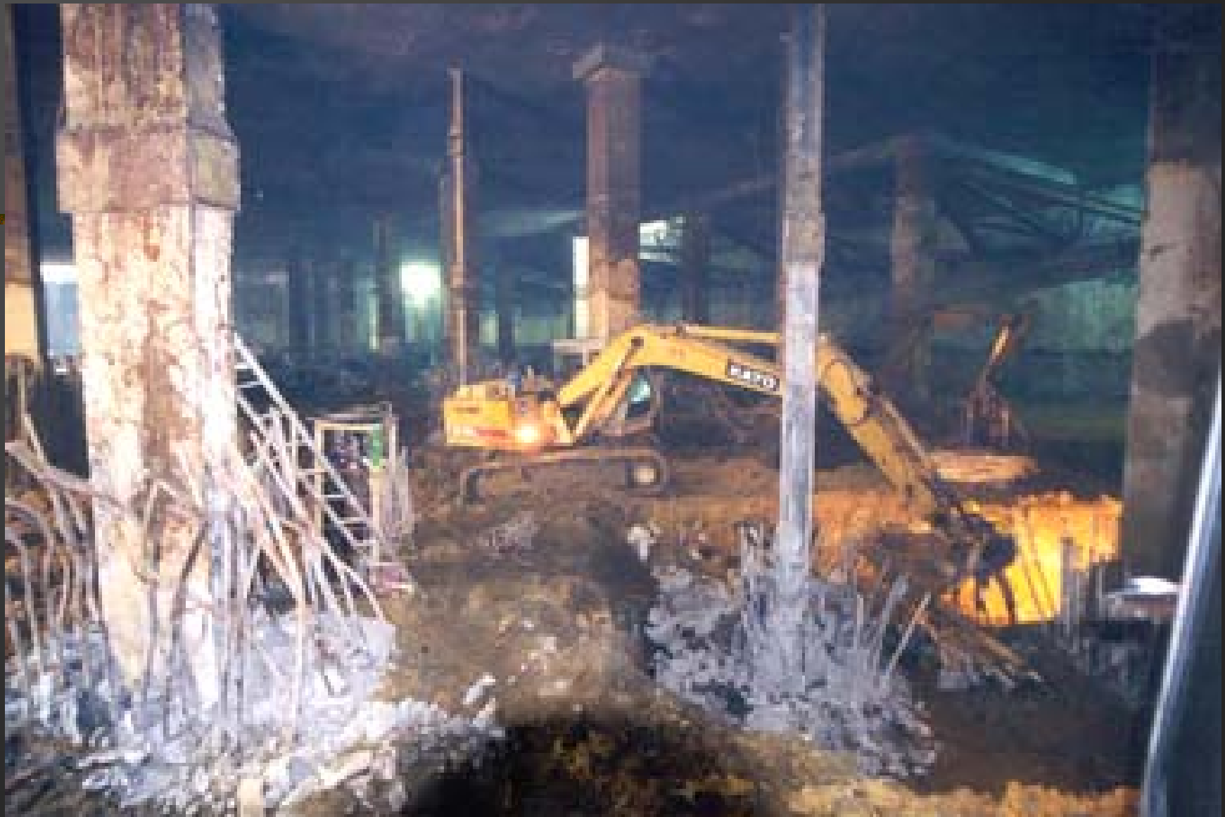
Excavation down to the formation level with pile head exposed
