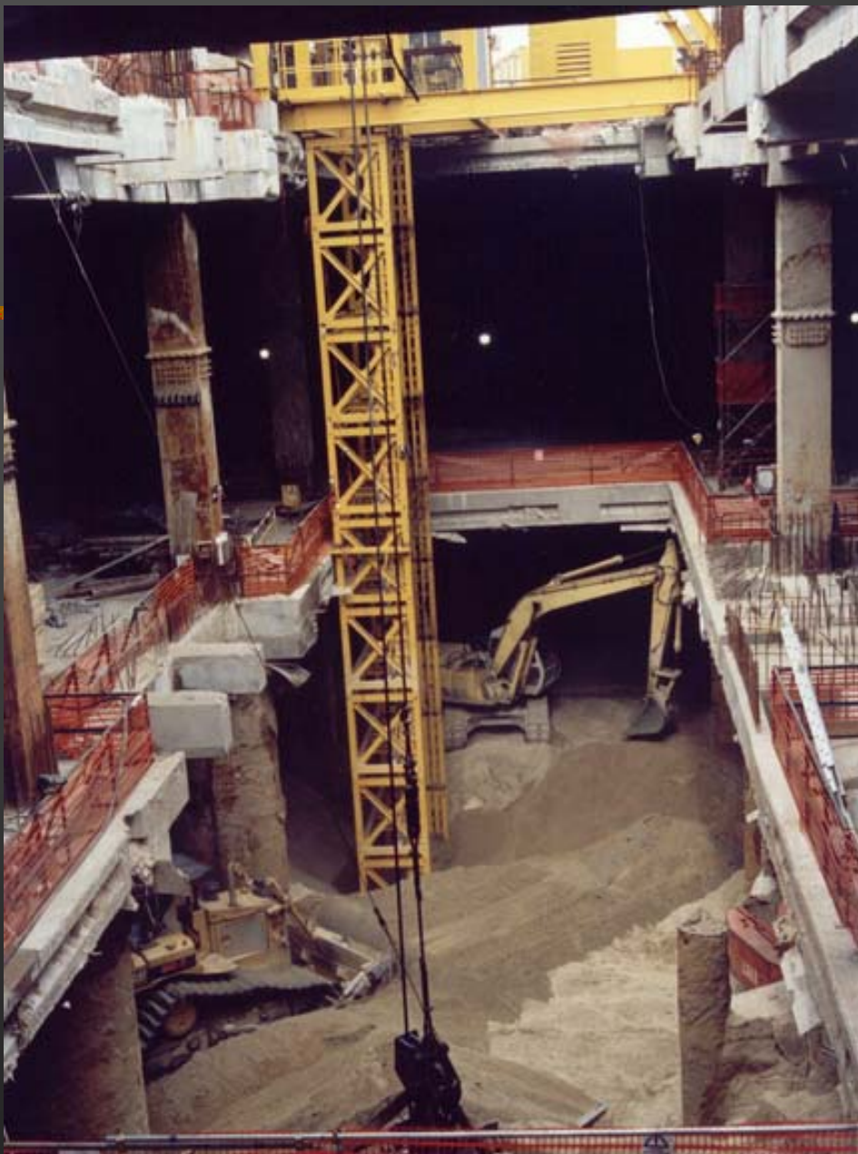
Excavation inside the basement
