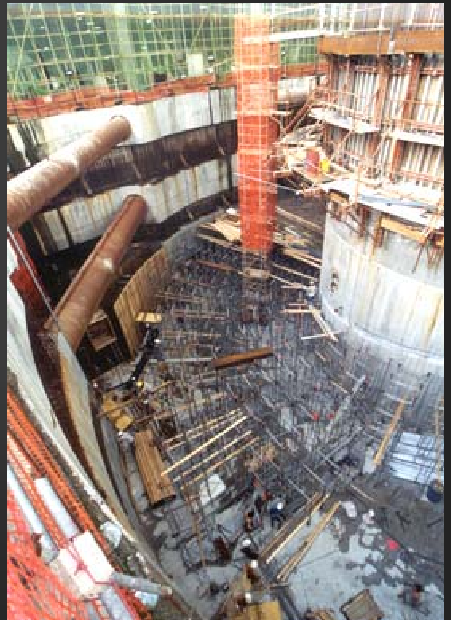
Forming the circular ramp
