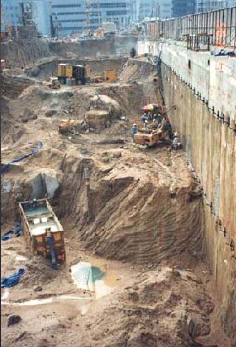
Forming the site and with diaphragm wall as the side support
