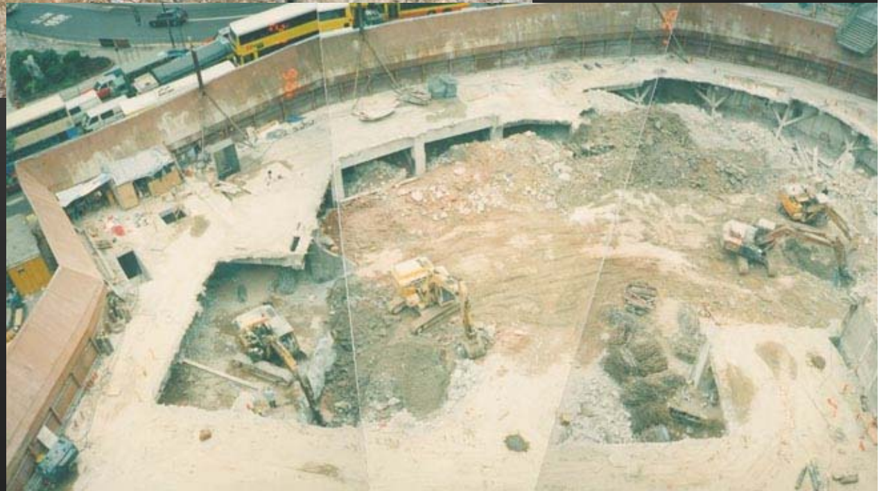
Demolition to the old Hilton Hotel including the 2-level basement structure
