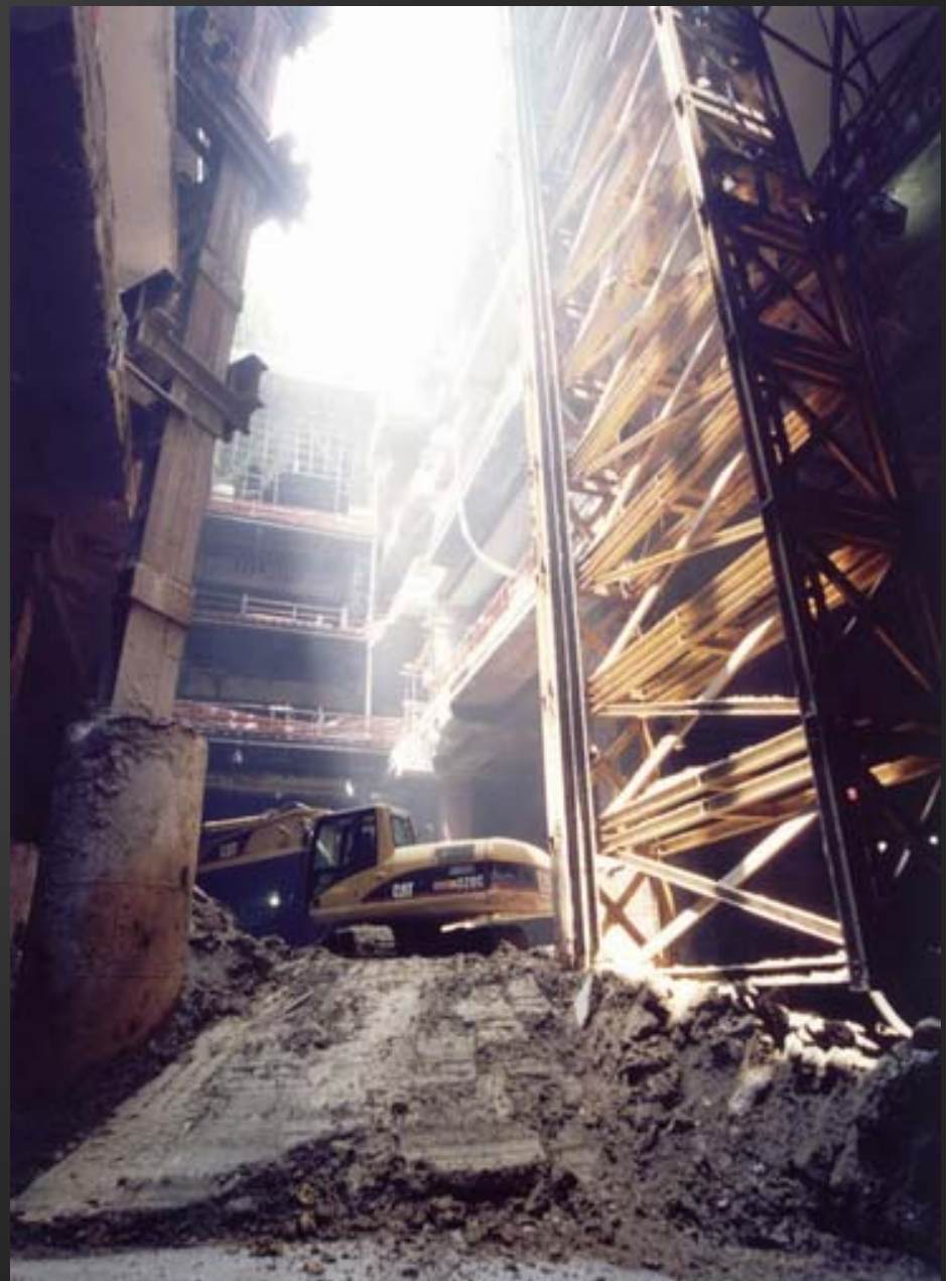
Excavation inside the basement
