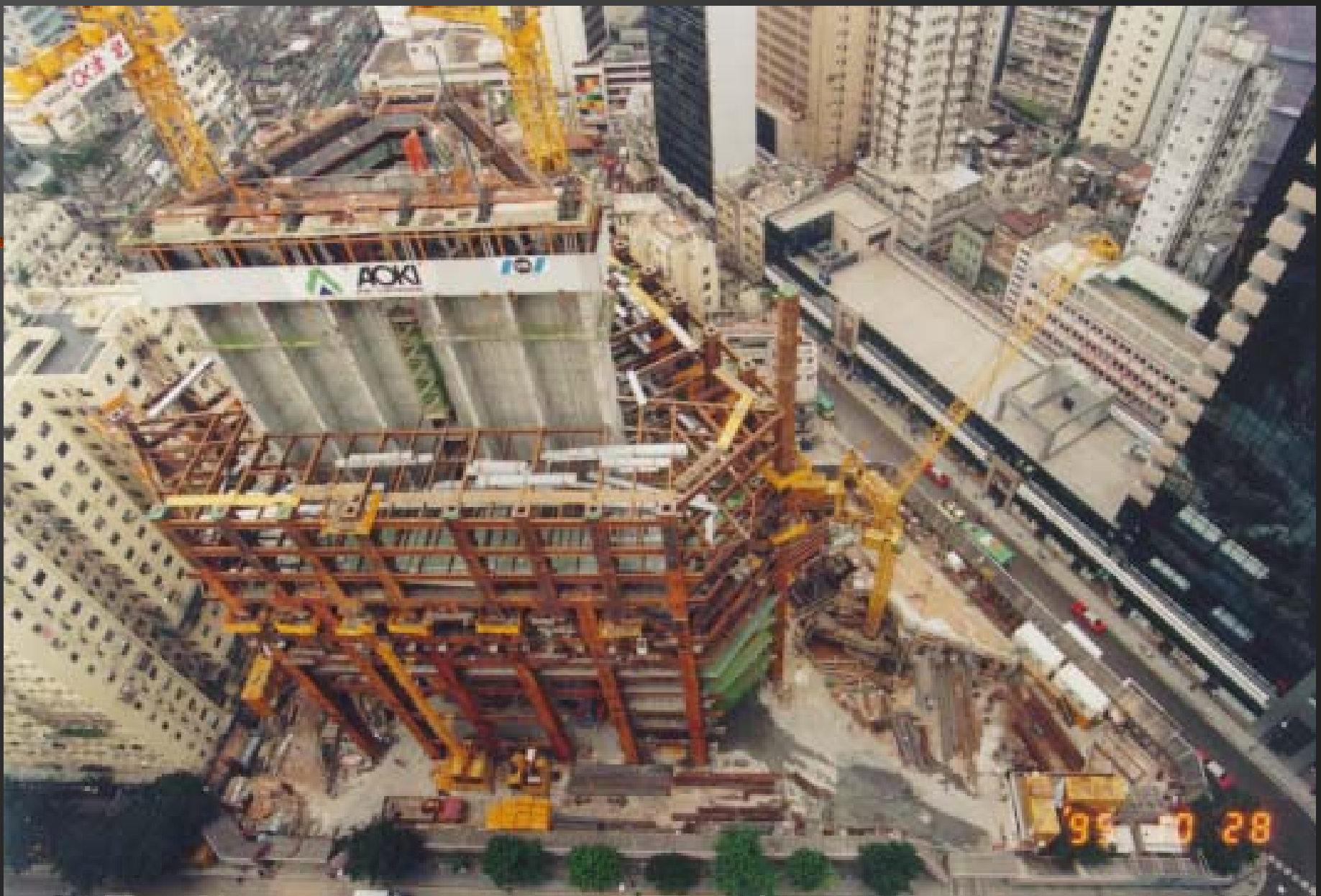
Superstructure and basement construction at the same time
