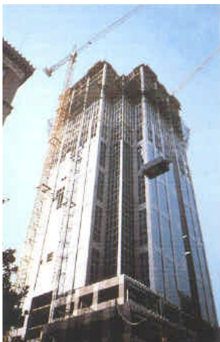
Fig. 2.1: Typical High-Rise Building under Construction
