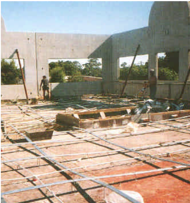
Fig. 2.8: ,Pecast Wall Panels
