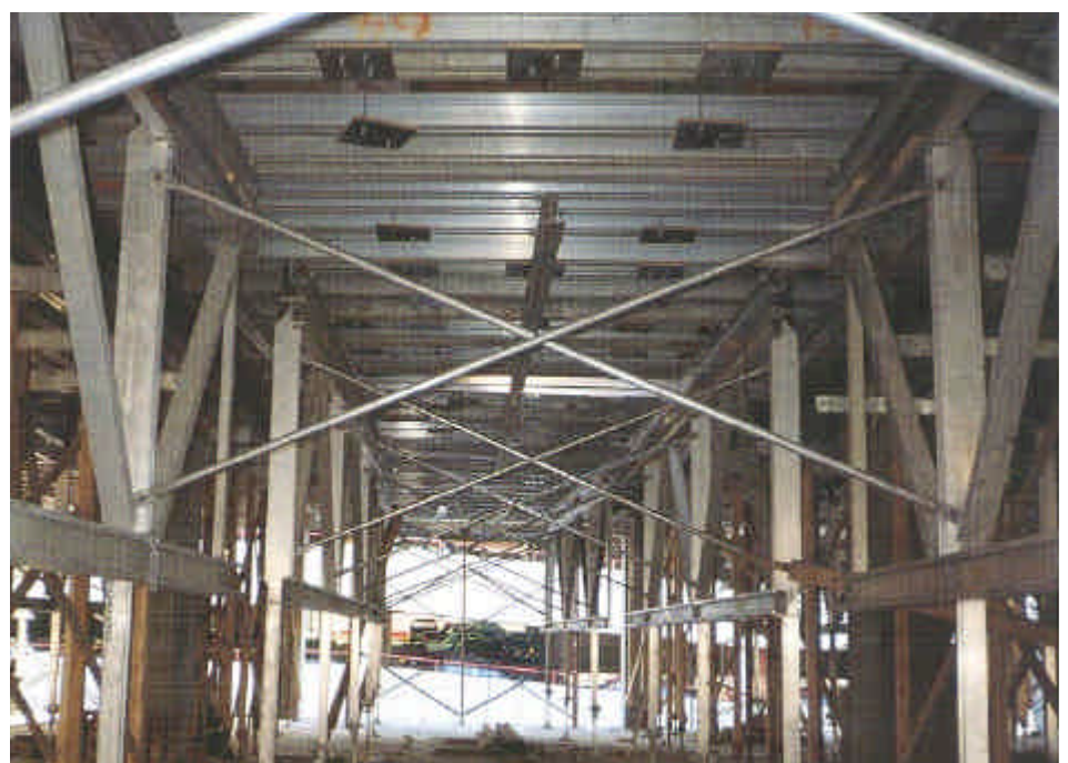
Fig. 2.4: "Flying Formwork" Panel Viewed from Inside of Floor under Construction
