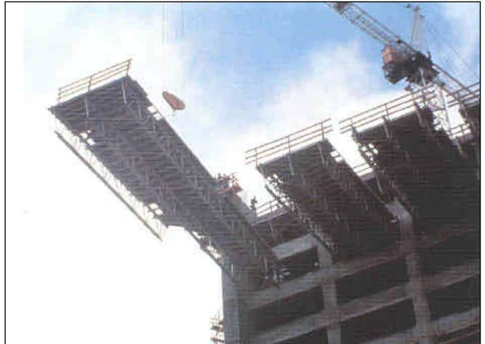
Fig. 2.3: Large "Flying Formwork" Panels
