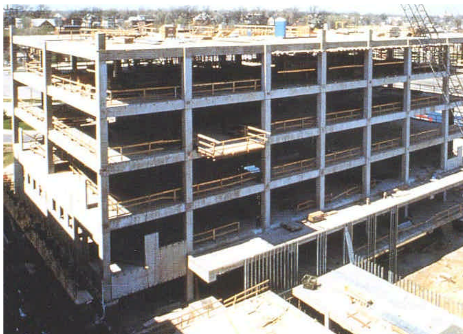
Fig. 2.2: Typical Low-Rise Building under construction
