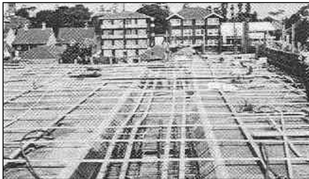
Figure 87: Positioned cables
