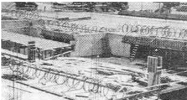
Figure 82: Scaffolds at construction joints with rolls of tendon
