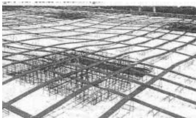
Figure 102: Cables in column region
