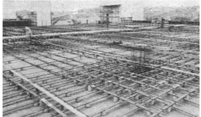
Figure 77: Flat slab during construction
