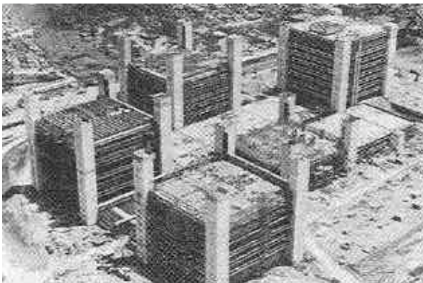
Figure 78: The Centro Empresarial during construction
