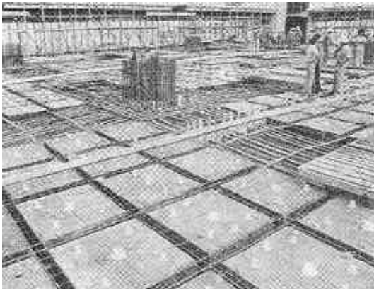
Figure 76: Waffle slab during construction
