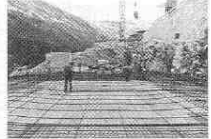
Figure 48: Supporting of tendons
