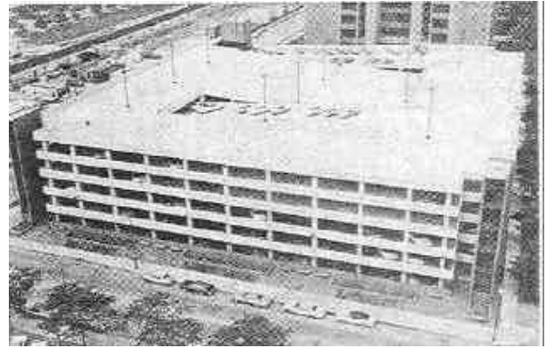
Figure 13: Multi-storey car park
