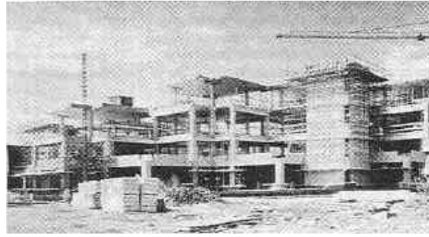
Figure 91: The building during construction
