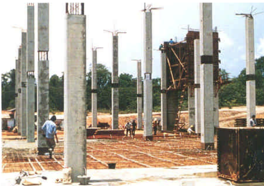
Fig. 2.7: Another Example of Efficient Construction: 2-Storey Pre-Fabricated Concrete Columns
