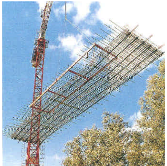
Fig. 2.6: Site Pre-Fabricated Reinforcement, Including Strand and Anchorages, Speed up Construction
