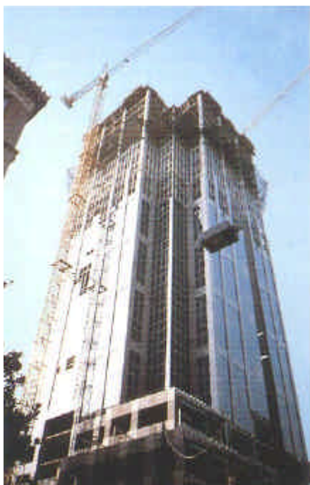
Fig. 2.1: Typical High-Rise Building under Construction
