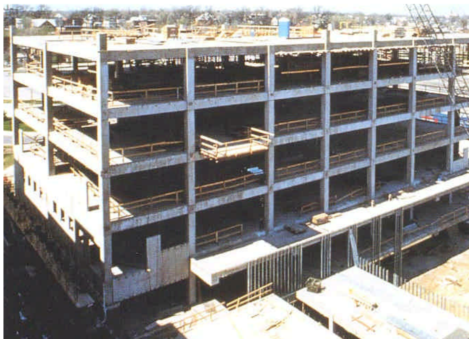
Fig. 2.2: Typical Low-Rise Building under construction
